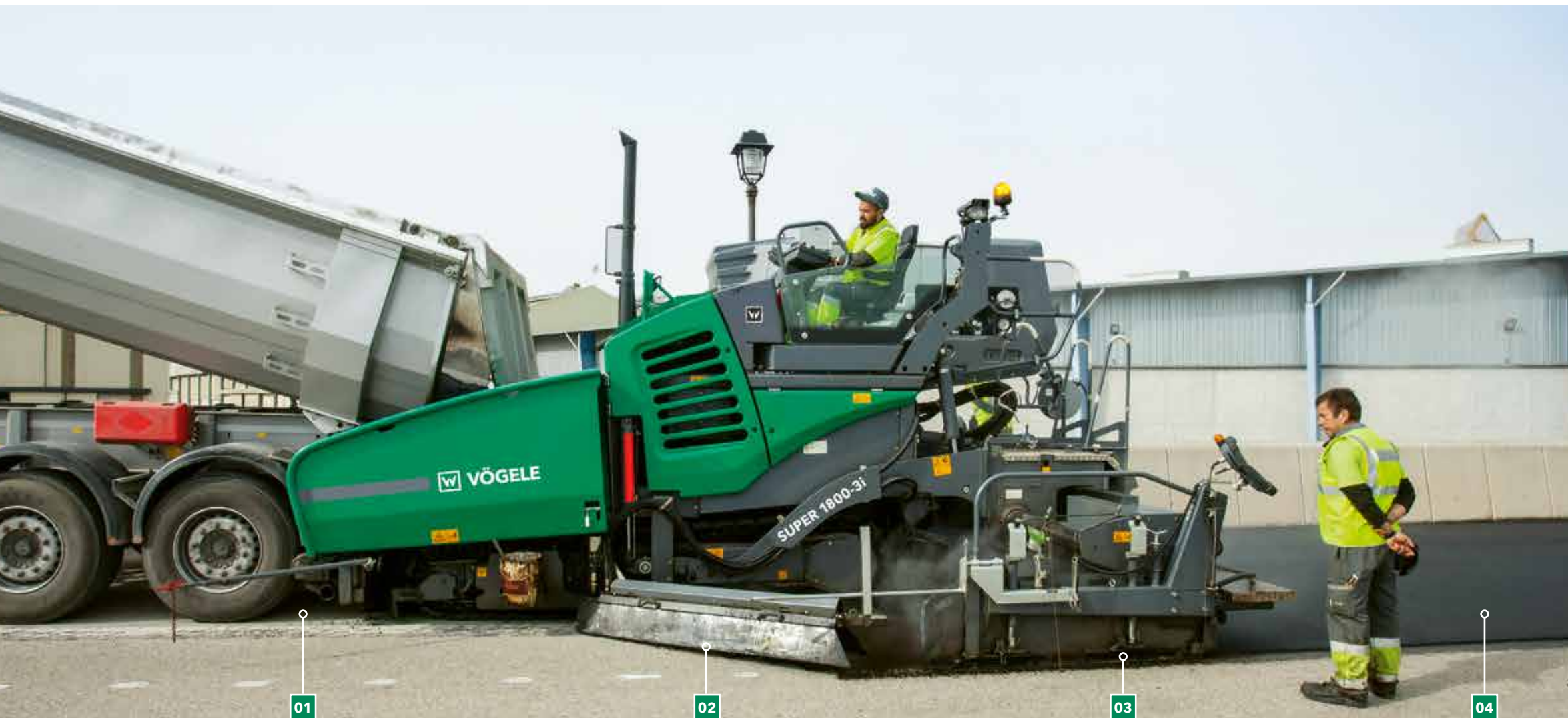
02 Hot bitumen emulsion at a temperature between 70 and 80 °C is applied by the spray paver.
