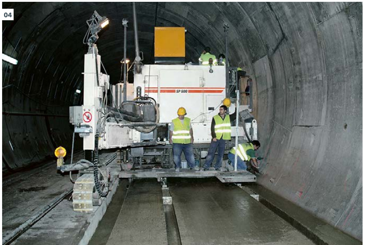
04 Zero-clearance paving below ground using stringless control.
