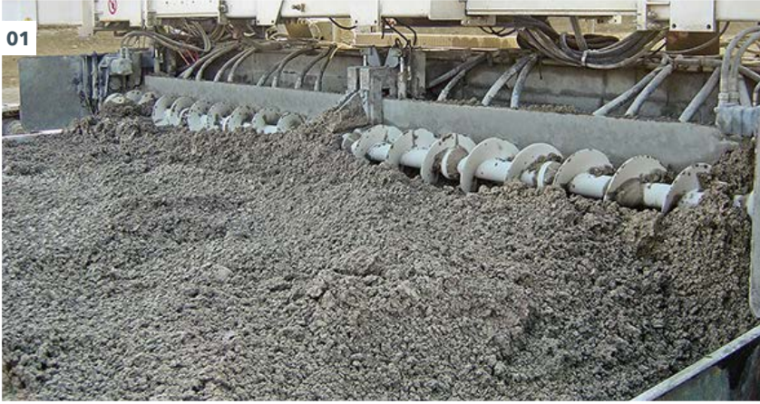
01 - 02 Inset application: spreading the concrete by means of a spreading auger or spreading plough.
