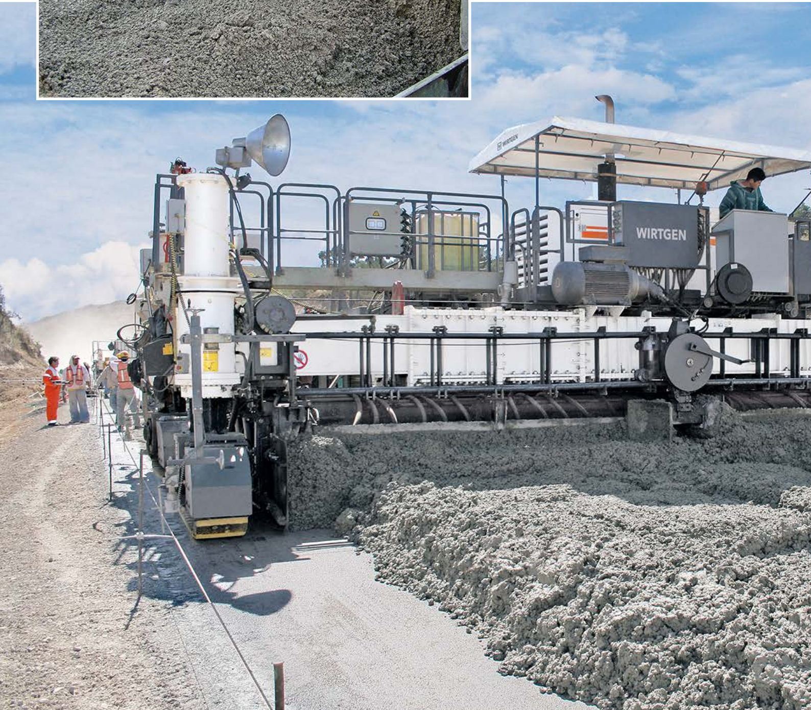
01 - 02 Inset application: spreading the concrete by means of a spreading auger or spreading plough.
