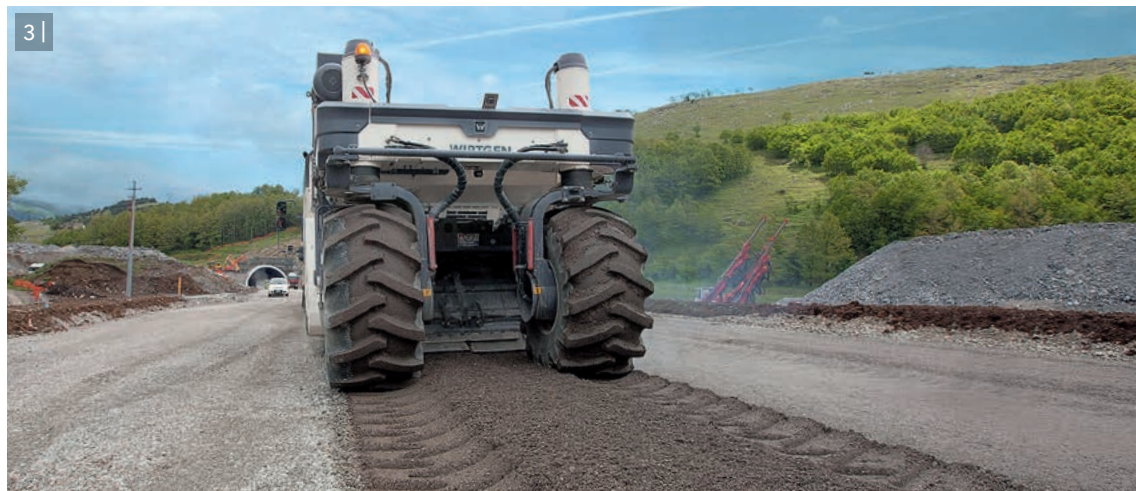
2-3 | Homogeneous asphalt mix processed by the cold recycler.
